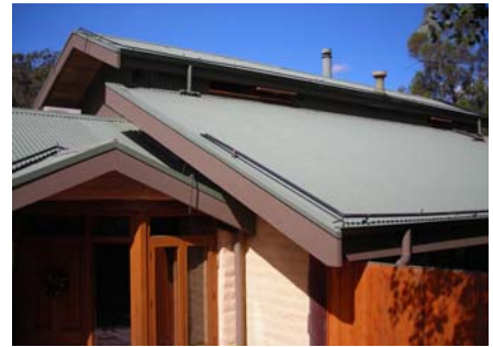
A pitched sloping roof minimises the chance of embers being trapped.
