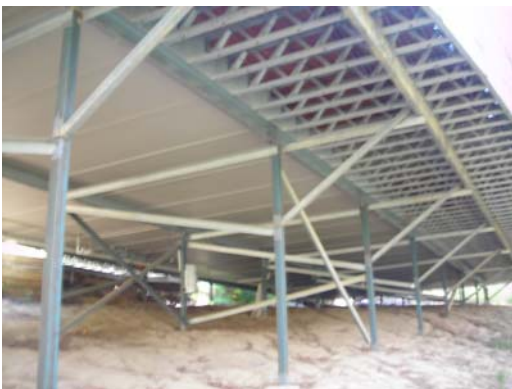
The decking boards on this verandah have no gaps to allow the passage of embers. Further protection is obtained through keeping the area free of vegetation.
