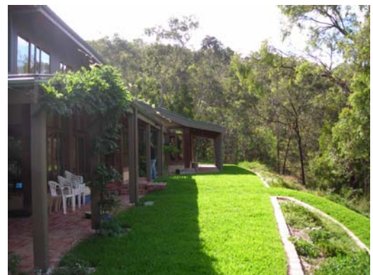
A grassy embankment, or "green vegetation zone", is a safe alternative to a verandah.
